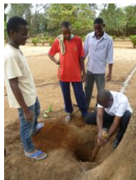
Digging the holes for the poles
